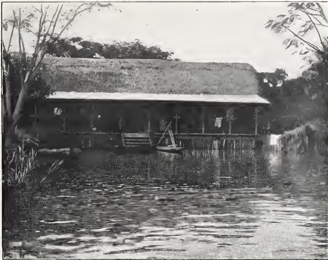
MONSEMBE STATION IN FLOOD
